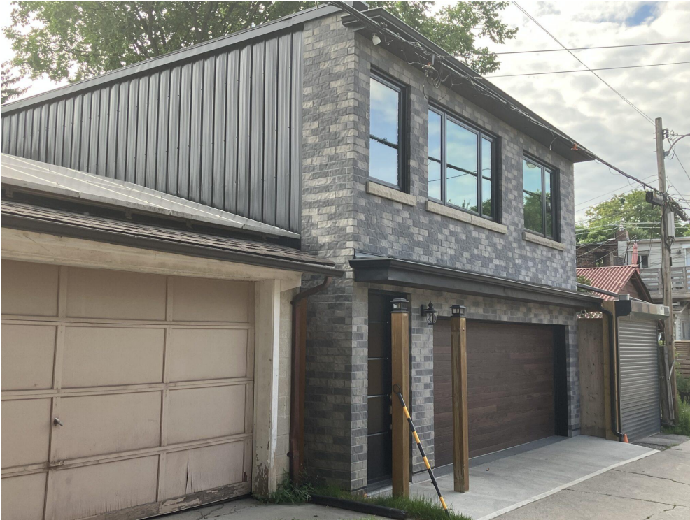
A new west side laneway house with interior parking
