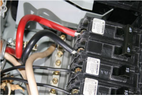
Aluminum wiring is the main wiring
